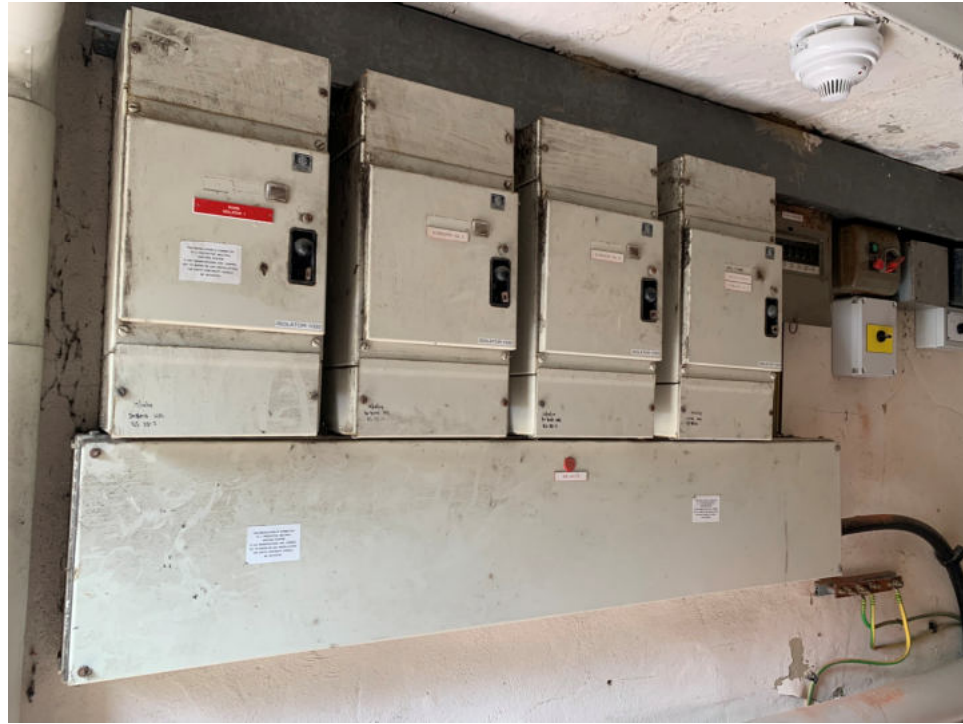
North Block Main LV Switch Panel
